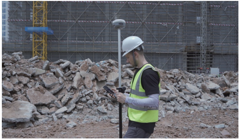
Surveying with Eyr RTK
